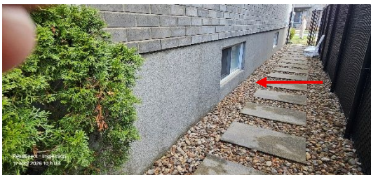
Earthworks and landscaping Negative slopes Left side
