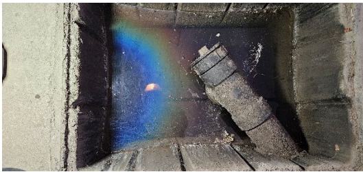
Retention pit - Gravity drain No major anomalies Garage
