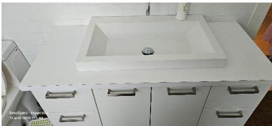
Cabinets and countertops (1) No major anomalies Bathroom
