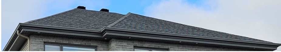
Roofing – Asphalt shingles No major anomalies Front facade
