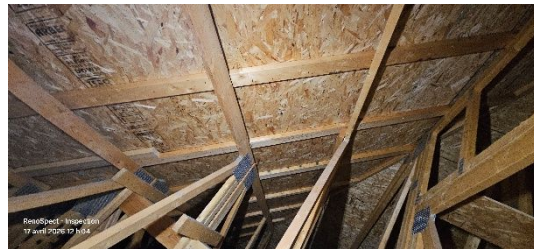
Decking No major anomalies Attic
