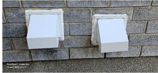
VRC – External Registers No major anomalies Right side
