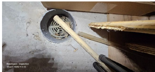
Floor drain No major anomalies (Mechanical chamber)
