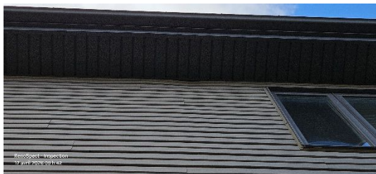
Soffits No major anomalies Rear facade
