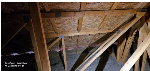
Attic - Thermal insulation and ventilation No major anomalies
