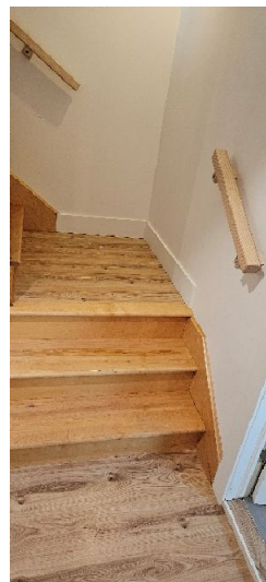
Interior staircases No major anomalies Basement
