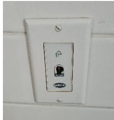
VRC – Switch No major anomalies Bathroom
