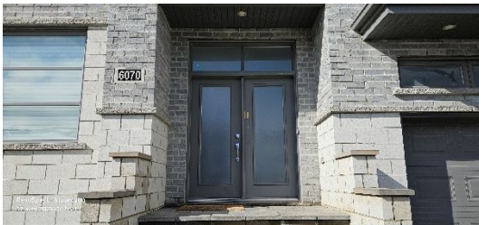
Front door No major anomalies Front facade
