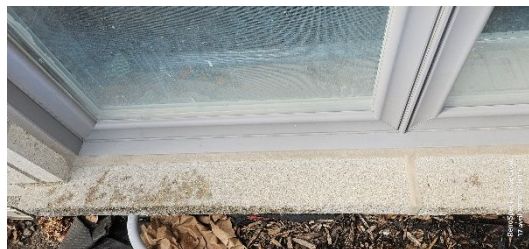
Sealant No major anomalies Front facade
