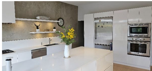
Cabinets and countertops (2) No major anomalies Kitchen
