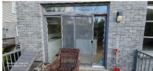
Patio door No major anomalies Rear facade
