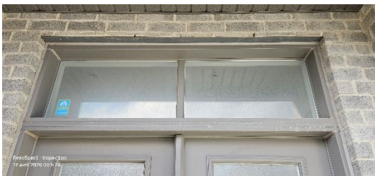
Sealant No major anomalies Front facade
