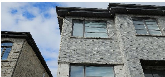
Exterior windows No major anomalies Front facade
