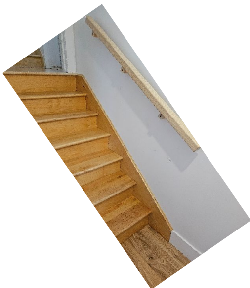
Interior staircases No major anomalies Towards the 1 st floor
