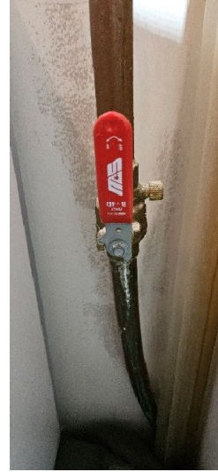
Water inlet (valve) No major anomalies Basement
