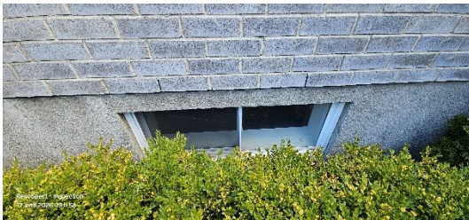
Earthworks and landscaping Presence of trees Rear facade
