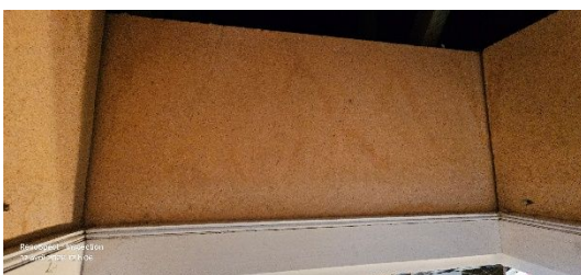
Attic - Access hatch Walk-in closet, 2 nd floor
