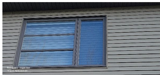
Exterior windows No major anomalies Front facade
