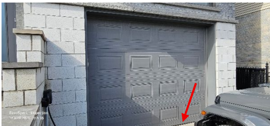
Garage Door – Maintenance (Air Vents) No major anomalies Front facade
