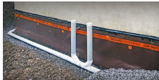
Example - Delta MS Membrane Typical installation
