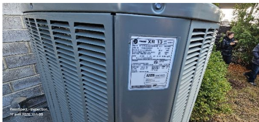
Air conditioning units / heat pumps (2) No major anomalies Rear facade
