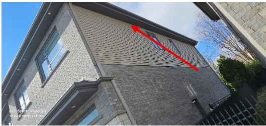
Aluminum clinker Deformation Right side
